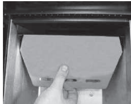
Pict. 16: Rotate the fire shield
