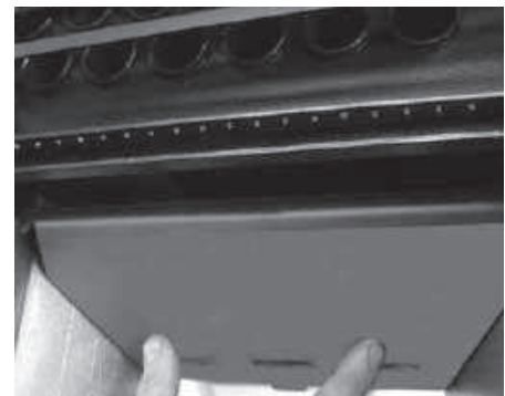
Pict. 14: Lift the fire shield
